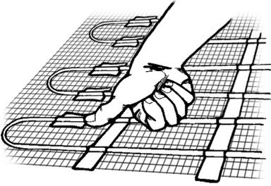
1. Recess the probe flat onto the floor approximately 50mm from the heating element. This is to ensure that it obtains the correct temperature readings. Use hot glue to hold it in place.
