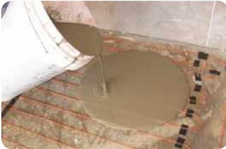
Using a flat trowel spread the leveling. It should be very easy to push and will find its own level. To protect the cable ensure you only move the trowel along the cable and not across it. You can use the top of the cables as a guide for the depth. The outline of the cables will be visible in the finished product.
