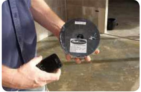
It is a good idea to cut a jig to the size you need it rather than use a tape measure the whole time. A off cut of wood is fine, in the picture we used an off cut of electrical cable.
